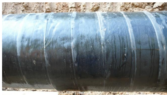
Figure 3. Appearance of the coating insulation based on LIAM tape. Gas pipeline branch in Kamensk-Uralsky DN 700
